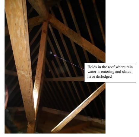
The rafters have been repaired in a few locations – again probably at the last renovation works. I note that there is a considerable extent dry rot near the base of the common rafters to the extent where lumps can be pulled out of the rafters by hand with little effort. The timberwork throughout the roof was found to have a heavy infestation of
