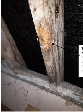
Typical example of dry rot present in many of the rafters in the roof. Very little structural integrity left in this rafter as lumps can easily be pulled out by hand. The Kingpost trusses and Purlin were stripped of paint with a layer of the outer surface hacked off. This was probably done to facilitate protim treatment for woodworm at the last renovation.
