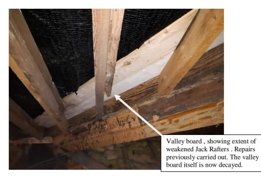
The photo above shows the underside of the valley where leaks regularly occur. The timber here is in an advanced state of Decay. Previous repairs show the extent to which the rafters had to be cut back. A similar process would have to be carried out on many of the rafters along the wallplate level of the roof.
